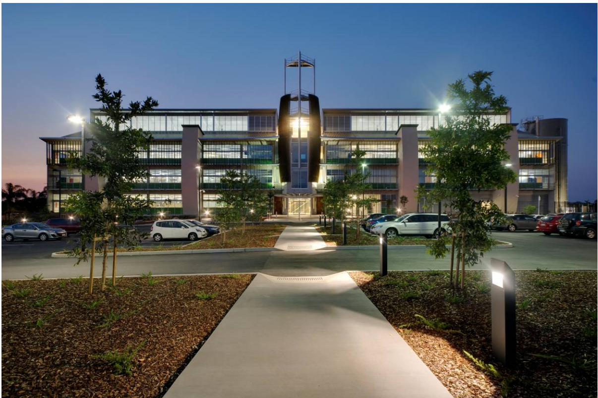
DCC Main Entry
